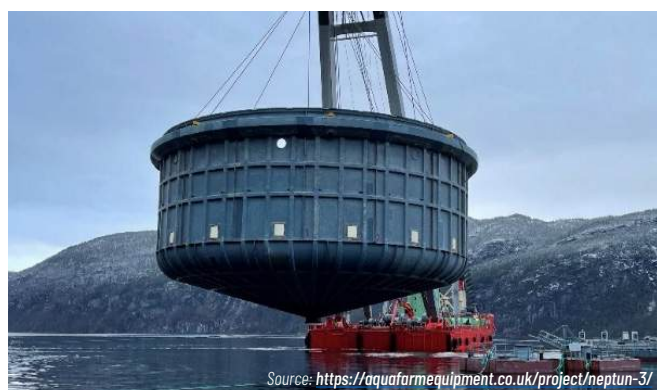
Figure 2: Neptun 3 semi-flexible containment tank
