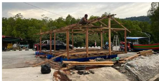
Constructing the oyster rafts
