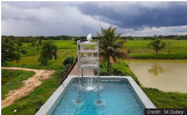
Aeration tower – a simple innovation of the project that solves the water quality problems in the hatchery
